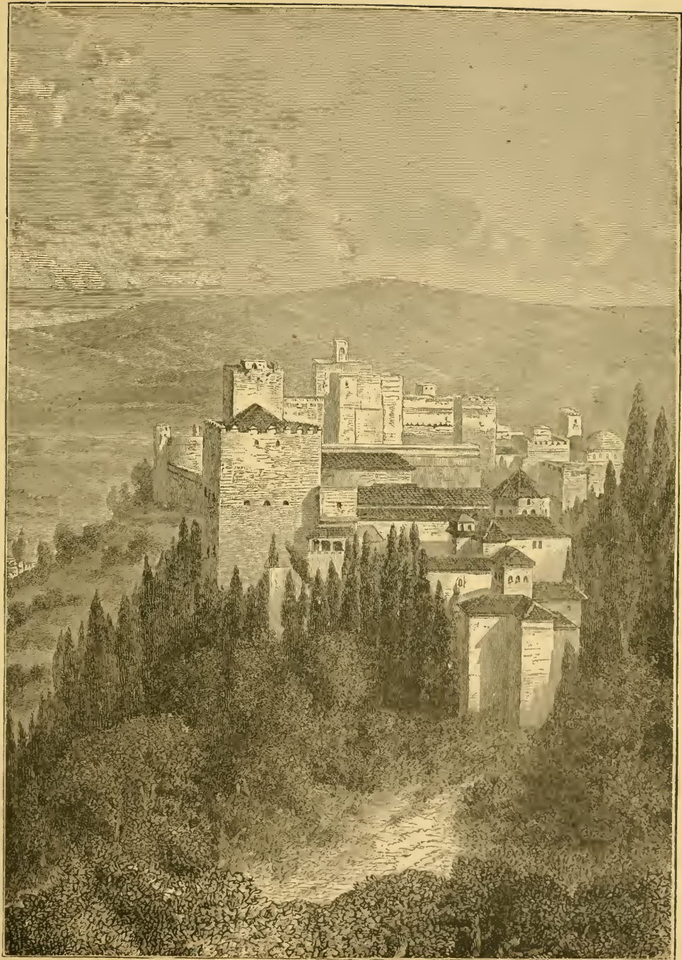
GENERAL VIEW OF THE ALHAMBRA.
